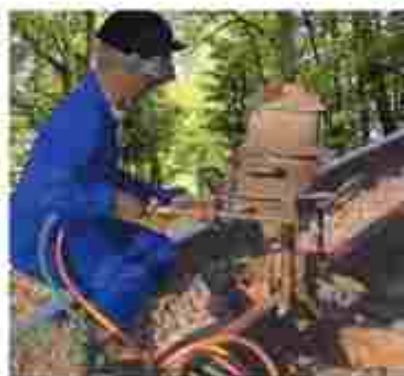
Figure 3.11 Thermite process for joining railway tracks
